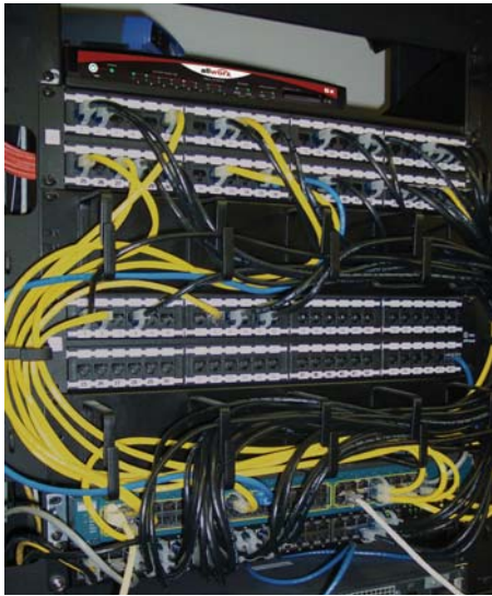
The Allworx 6x is shown above connecting to the Internet and PBX phone system to create the hub for Patrick Motors communication system.
